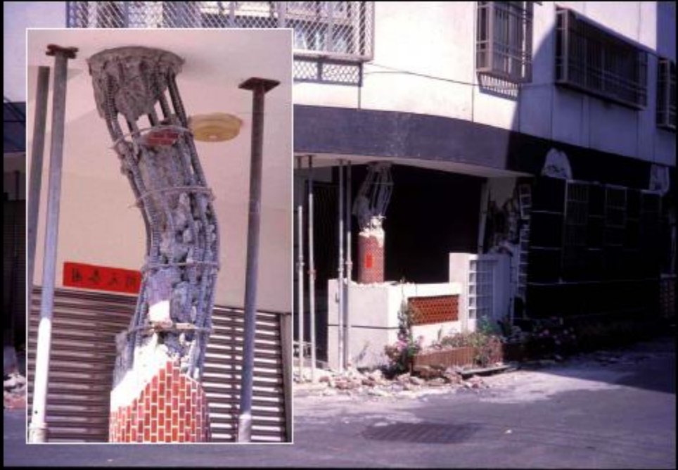
Brittle Shear Failure of Supporting Columns (Chi Chi EQ, 1999)
