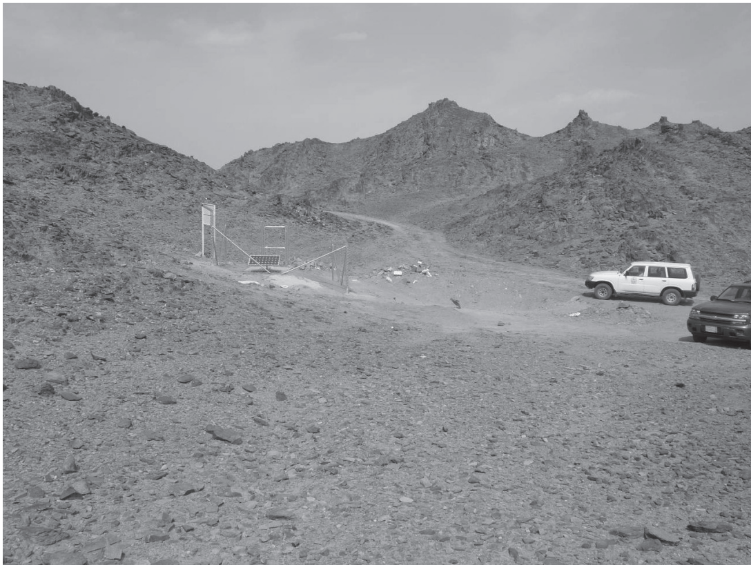
▲ Figure 2. Station sites were chosen for Precambrian bedrock contact. Site preparation included excavation to undisturbed bedrock with heavy equipment.
